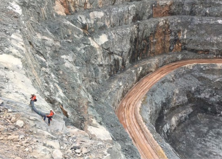
Enterprise Gold Mine, Rockfall Rockfall Drape Installation
